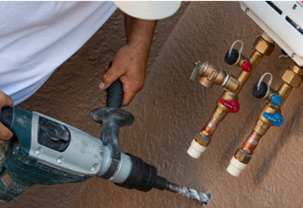
In temperate climates, installing a tankless water heater on an exterior wall can minimize installation costs.
